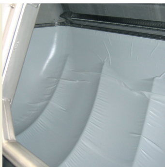
Spiral elements behind the membrane
